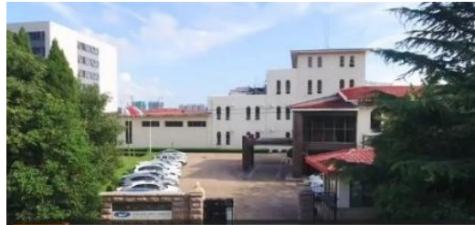
Qingdao Fuso Refining & Processing Co., Ltd.
