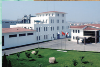
▲Qingdao Fuso Refining & Processing Co., Ltd.
